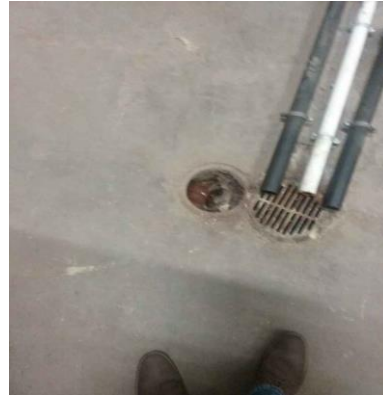
Missing cover drain. Creating trip hazard.
