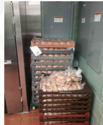
Blocked electrical panels.
