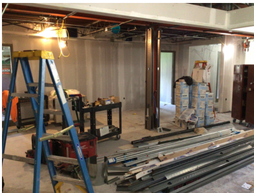
Central Ed. – Admin area drywall taping in progress.
