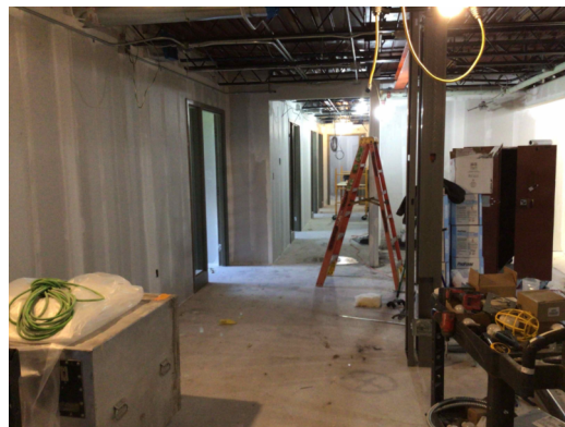
Central Ed. – Admin area drywall taping in progress.
